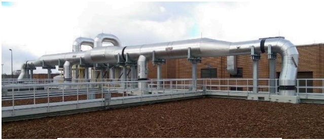
78,300 SCFM Biofilter Inlet Ductwork
