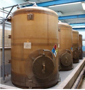
7' Ø Sodium Hypochlorite Tanks
