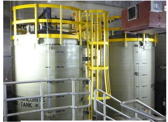
10' Ø Sodium Hypochlorite Tanks
