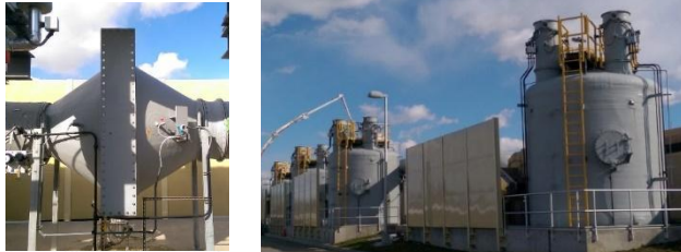
Four (4) Grease Filters and 14' Ø Dual Bed Carbon Adsorbers
