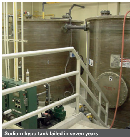
Sodium hypo tank failed in seven years
