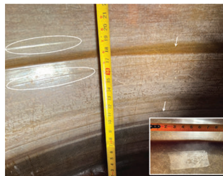
Figure 9. Imprinting of tank shell and bottom molds.
