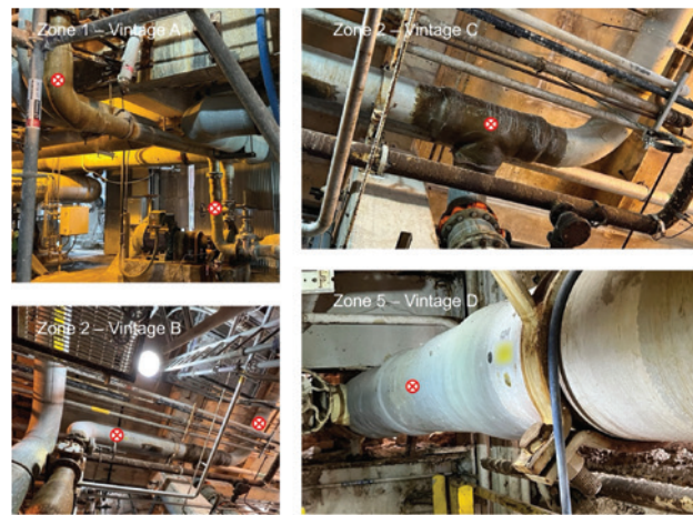
Figure 2. Single circuit with multiple pipe manufacturing vintages.
