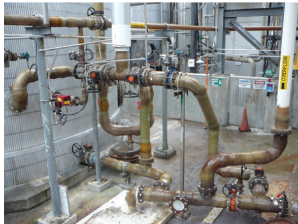
Figure 1. Chlorine dioxide piping.
