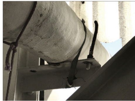
Figure 4. Improper pipe support.
