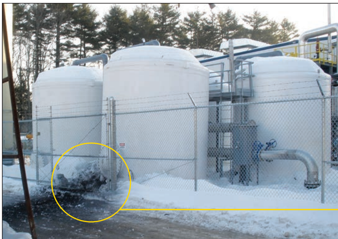
Photograph 1. A carbon absorber failed catastrophically within five days of startup, when the anchor system failed, and bottom blew out.
