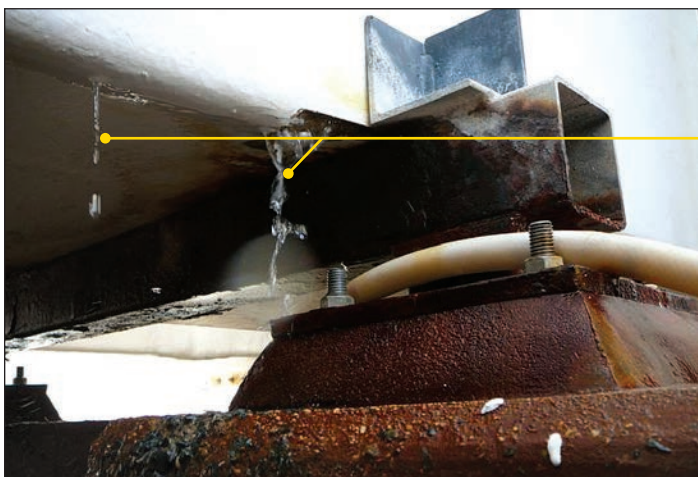
Photograph 4. Close-up of the cracked, leaking area of the vertical scrubber duct section.
