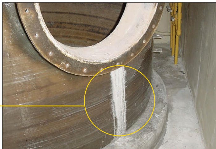
Photo 6. Close-up of FRP deterioration on one of the sodium hypochlorite tanks.
