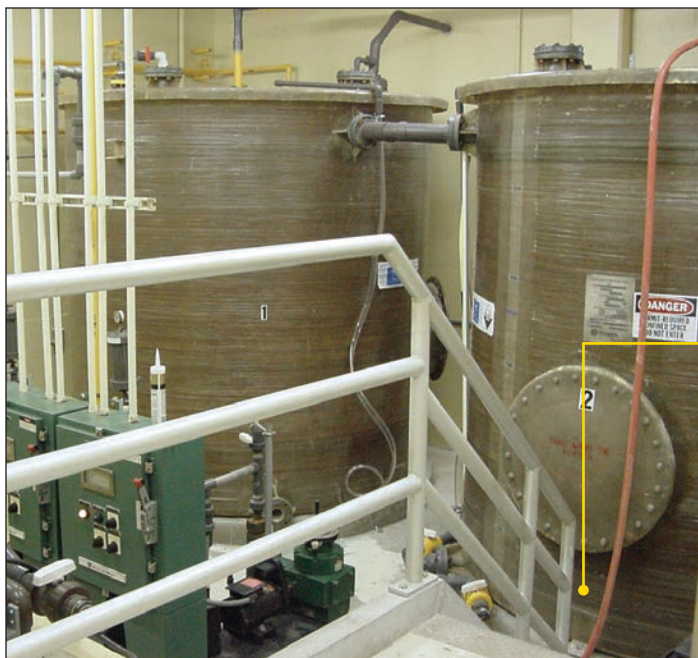
Photograph 5. Pair of sodium hypochlorite tanks that were replaced after seven years of service due to excessive FRP deterioration and through-wall leakage.
