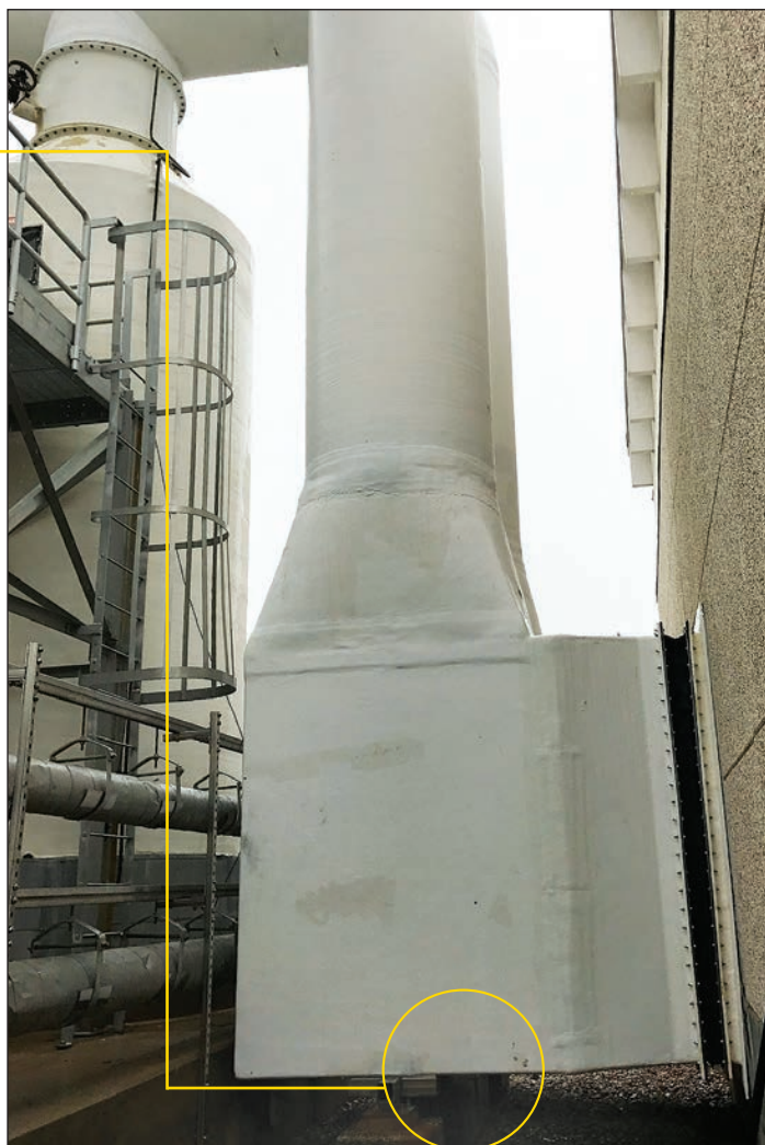
Photograph 3. A repaired vertical scrubber duct section that was improperly supported, cracked and leaked hazardous corrosive condensate.
