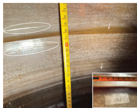
Figure 9. Imprinting of tank shell and bottom molds.
